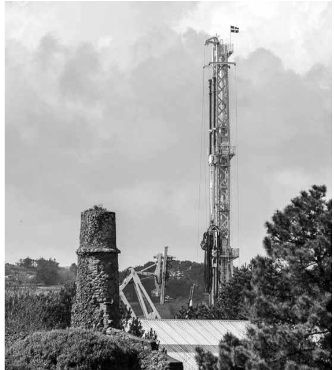
A geothermal drilling rig at United Downs, near Redruth, sits alongside an old Cornish mine chimney.
